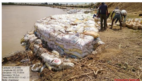
Mitigation of flood through a sandbag check dam at Chandpur village
